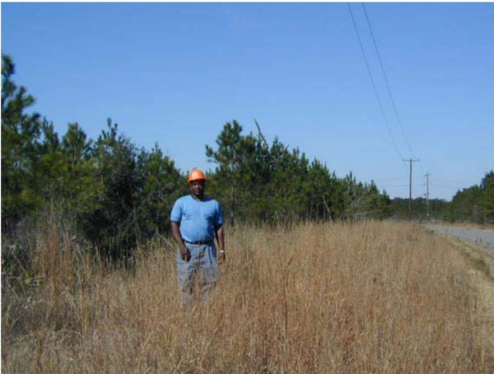
Photo 5. Good trimming under a single-phase line with three herbicide cycles
