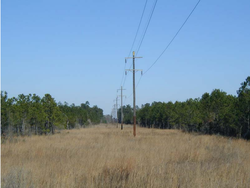
Photo 6. 69 kV right-of-way after three herbicide cycles
