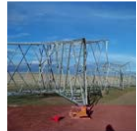
Transmission towers ready
