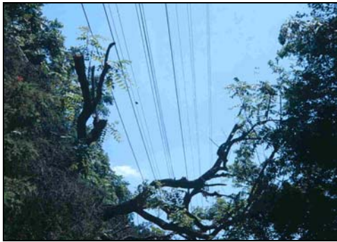
Directional pruning for line clearance
