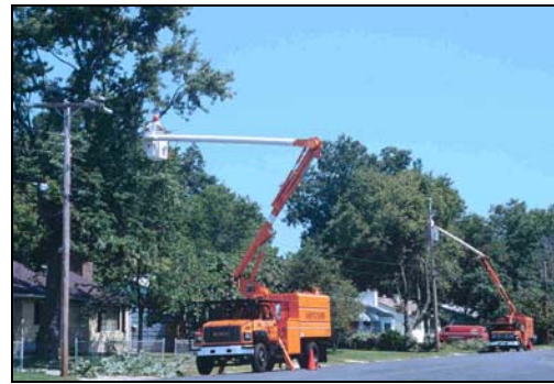
Trained arborists removing limbs in utility easements
